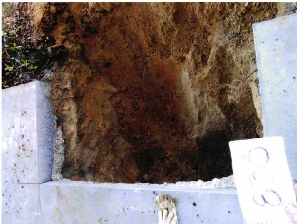
Picture 2: UST 835Azalea excavation.
